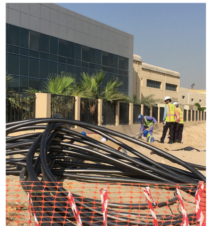
DEWA - Installation & Commissioning of 11kV Cables
