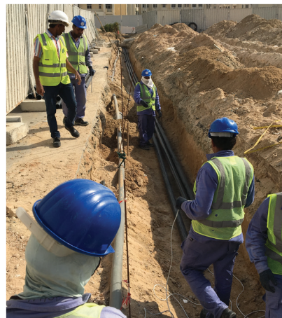
DU - Telecommunication Ducting Infrastructure Work
